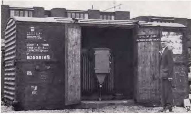
Mr. Mills at the temporary 'wagon' substation.
